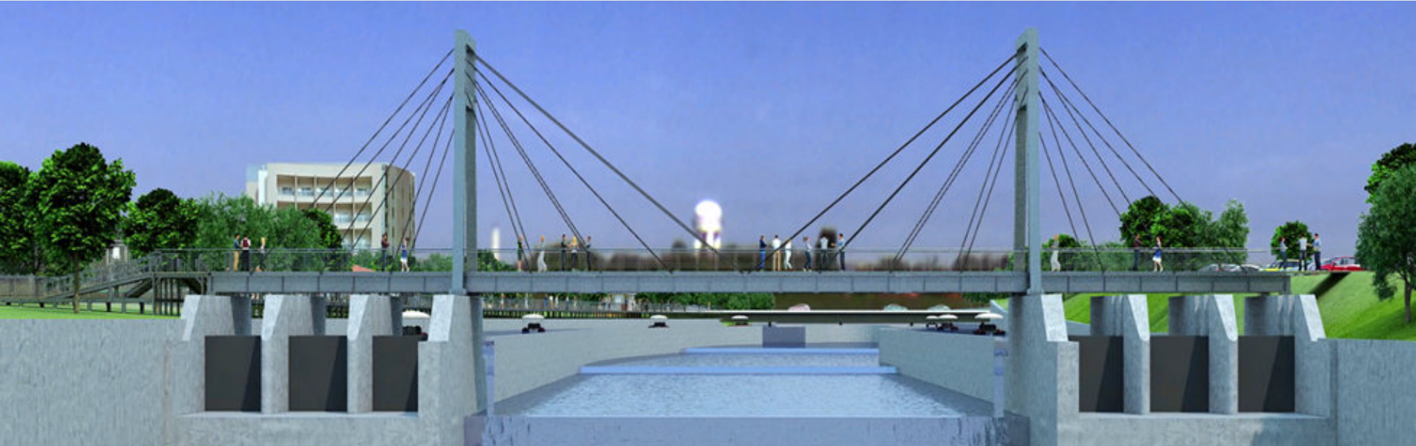
CAN PEDESTRIAN BRIDGE / CANAKKALE- 2017
